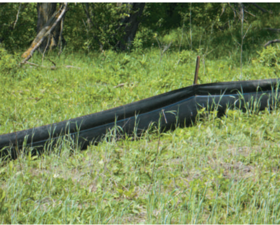
Figure 1.2 This technical textile reduces soil erosion on a slope.
